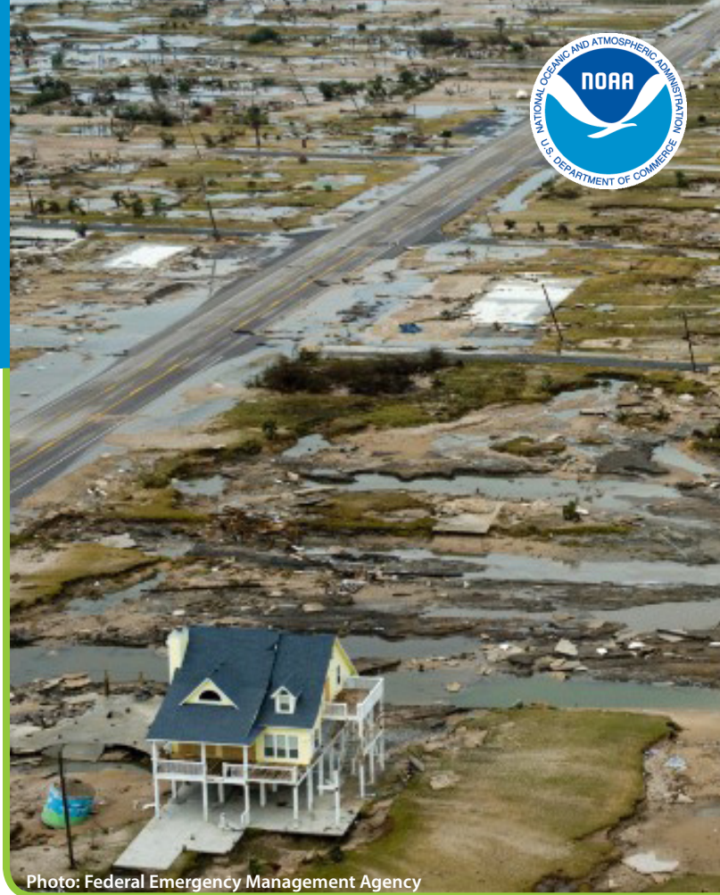
Photo: Federal Emergency Management Agency
