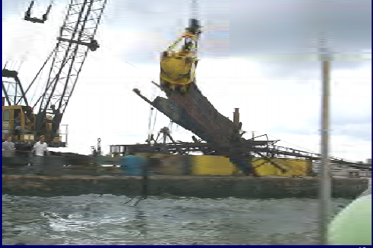
Typical Method of Derelict Vessel Removal
