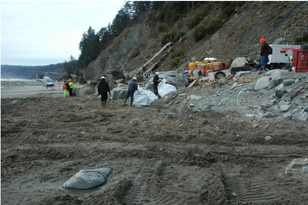
Figure 16: Site cleanup after dock removal is completed (Photo: The Undersea Company)
