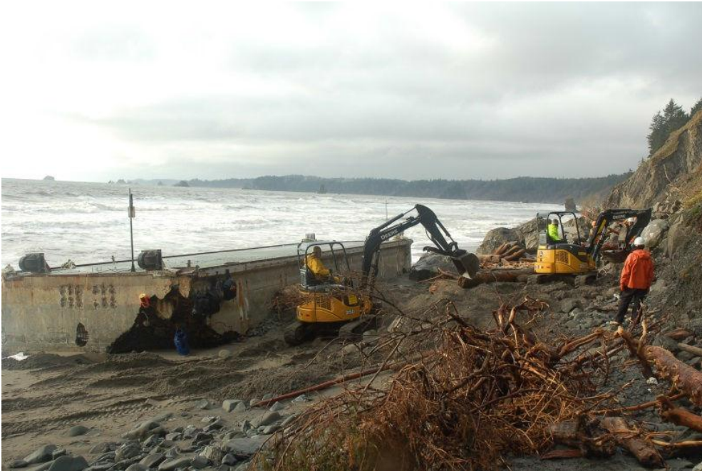
Figure 13: Mini excavators constructing the berm (Photo: The Undersea Company)
