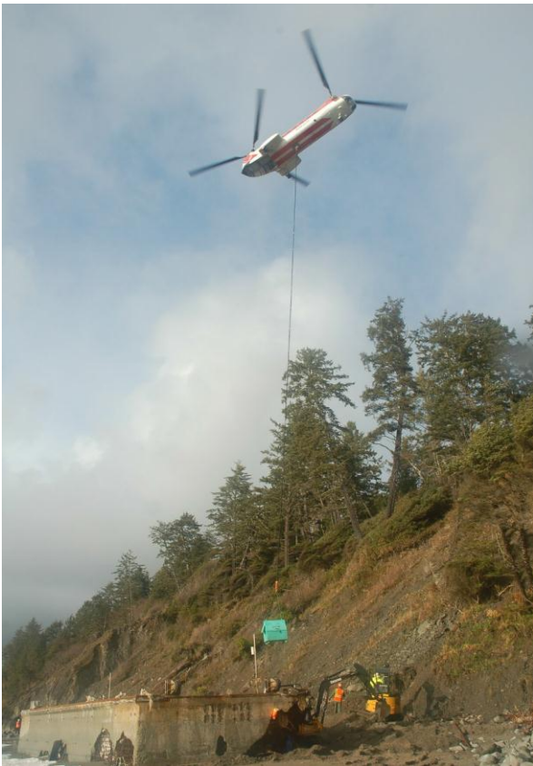
Figure 12: Mobilization of equipment with the Vertol helicopter (Photo: The Undersea Company)
